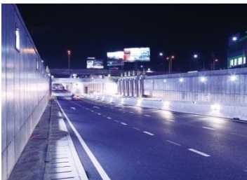
Street Lighting in Bangkok, Thailand
